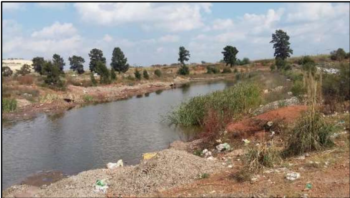
Photo 2: Stormwater run-off into excavated holes on the Libanon Landfill Site (2017)
