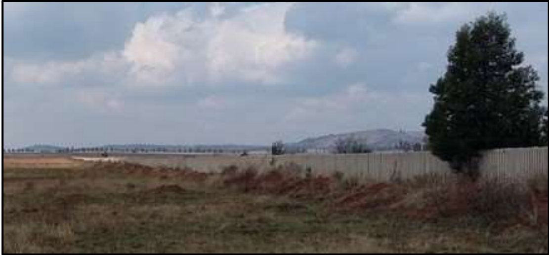
Photo 1: Palisade Fence on the Perimeter of the existing Libanon Landfill Site (2017)
