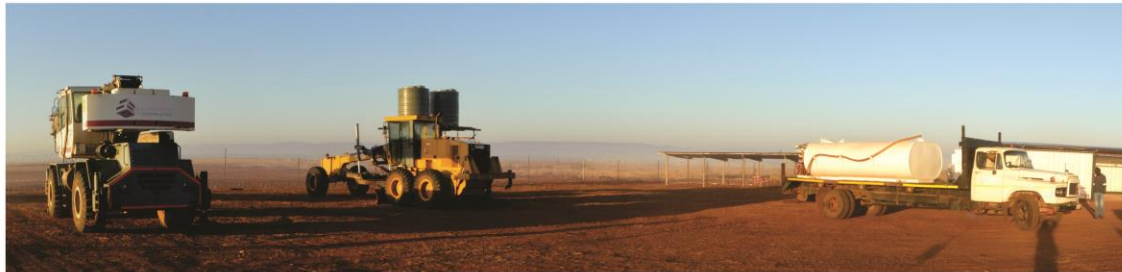
View 7 and 8: View of the construction camp site and equipment on site.
