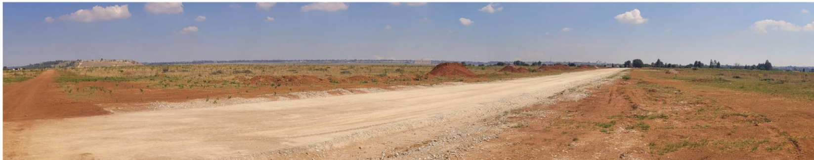
View 13: View of the temporary road that is now a properly constructed access road - 5 November 2025.
